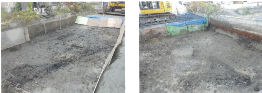
写 2-2.1 掘削側面養生状況
